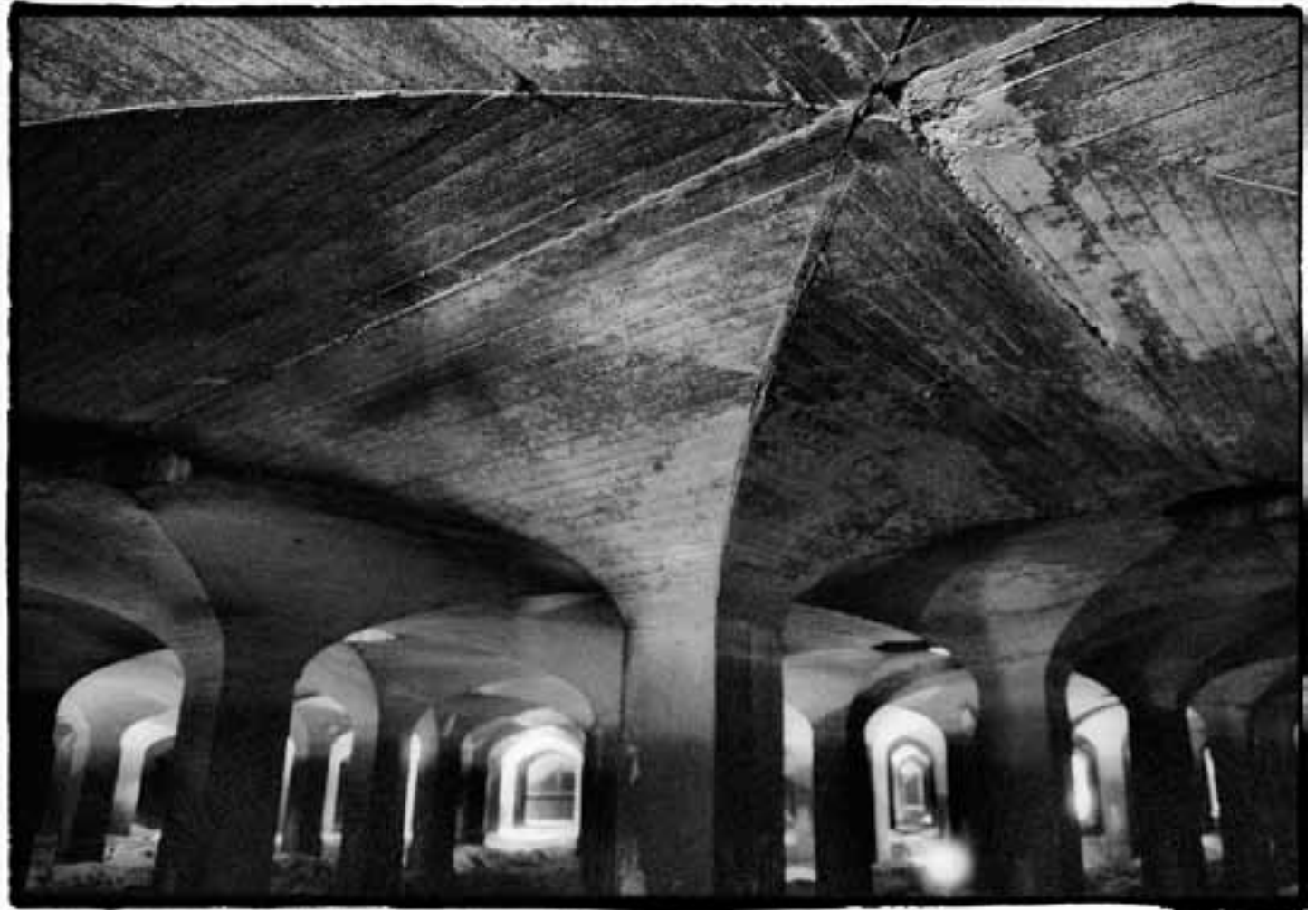
Disused water filtration facility.
