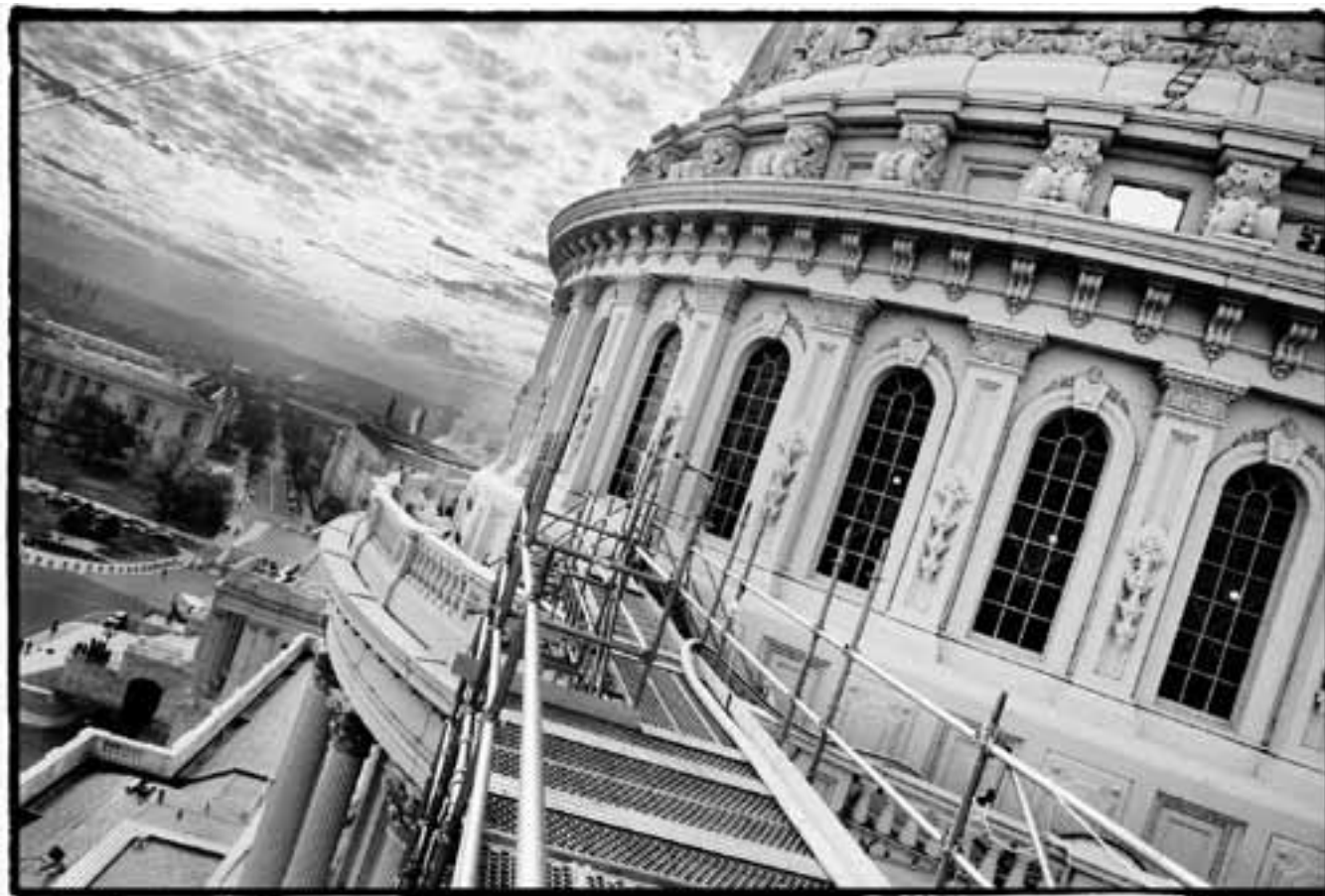
The US Capitol with catwalk scaffold
