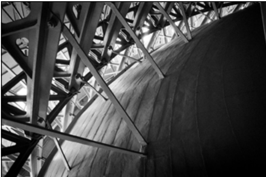
US Capitol Dome interstitial space
