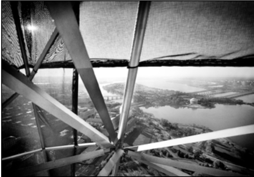
View to the Tidal Basin from the Washington Monument scaffold, 1999.
