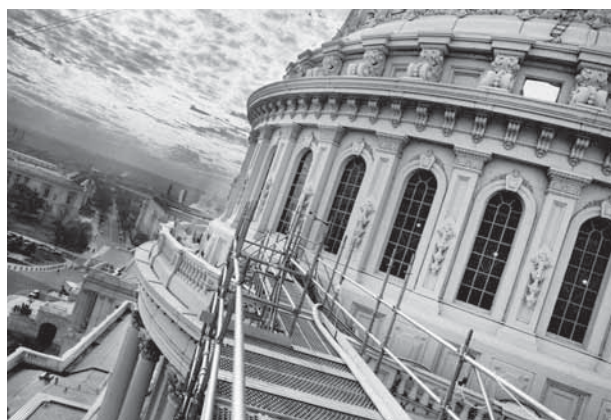
US Capitol with scaffolding
